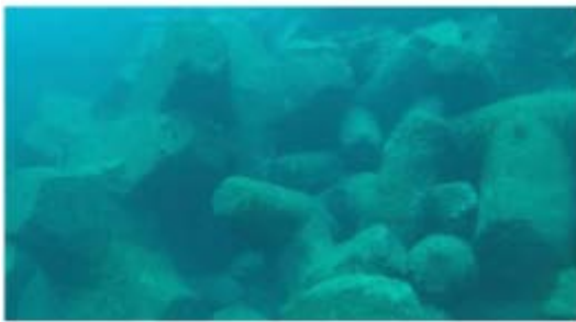
图6 K0+140m~K0+320m 扭工字块大量断肢
