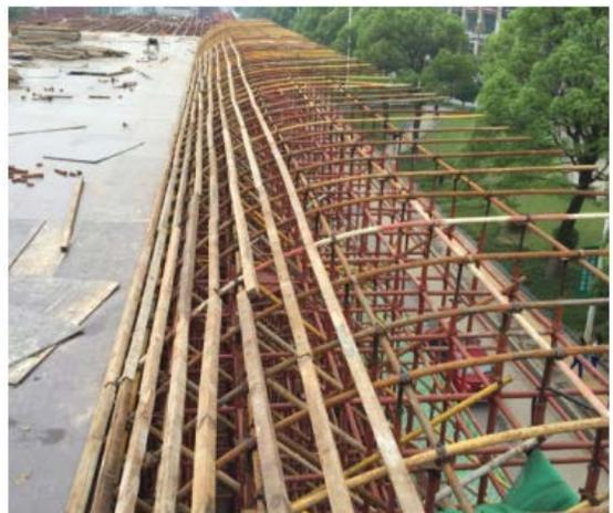
图3 侧模曲面异形脚手架搭设
